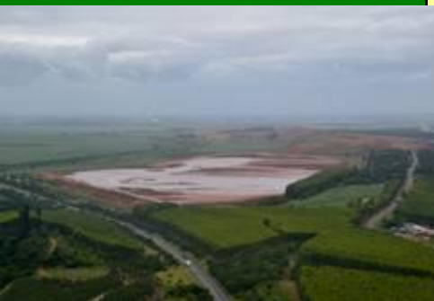
Slimes dam from south
