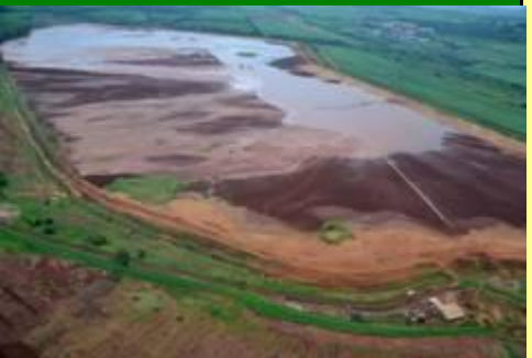
Slimes dam from the north
